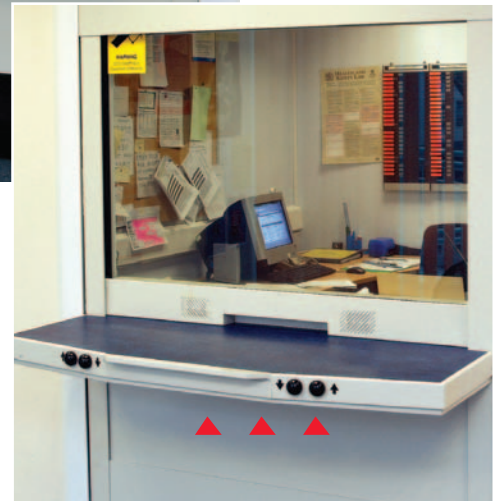
An obstacle detection system allows the counter to be raised or lowered without risk to the public.
